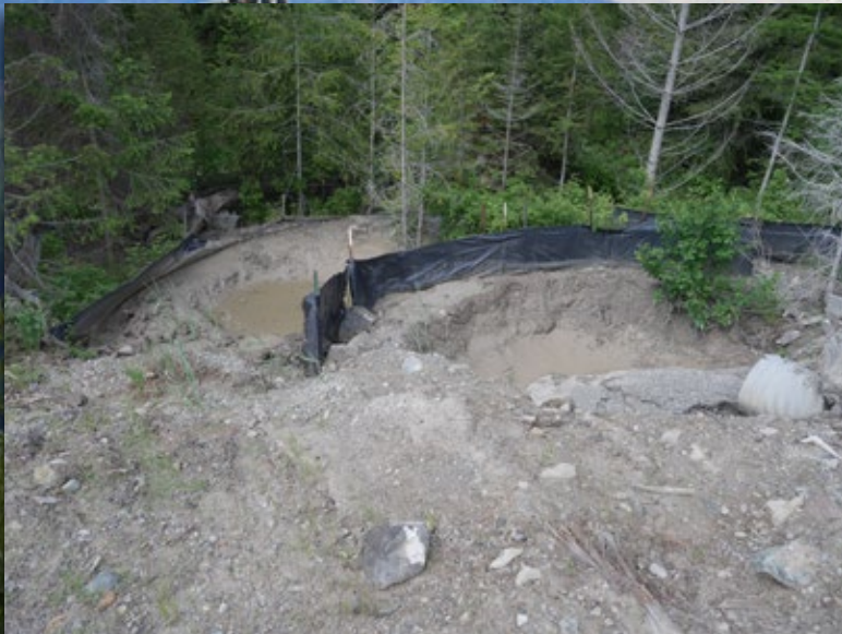
Where water runs off roads built for the mine, sediment -- loose silt, clay, sand, and other soil particles -- can get washed into waterways. Here, silt fences have been installed to help address the concentrated sediment release at a culvert.
