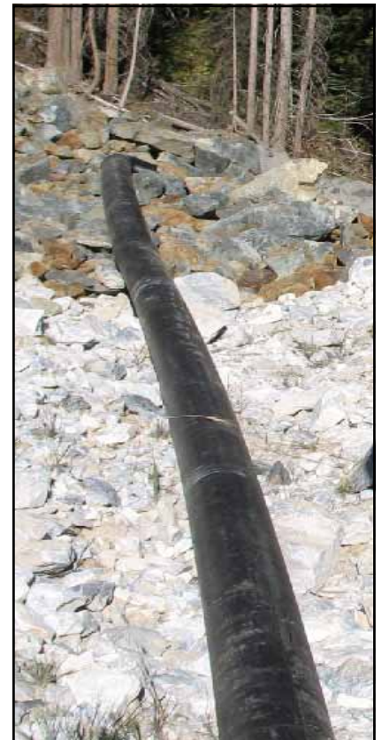
Pipe that was discharging treated mine water over the rubble above Gold Bowl Creek
